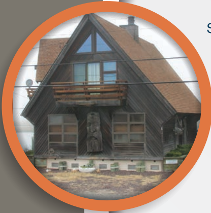
First Smart Vent installation in Avalon, NJ. 1999
